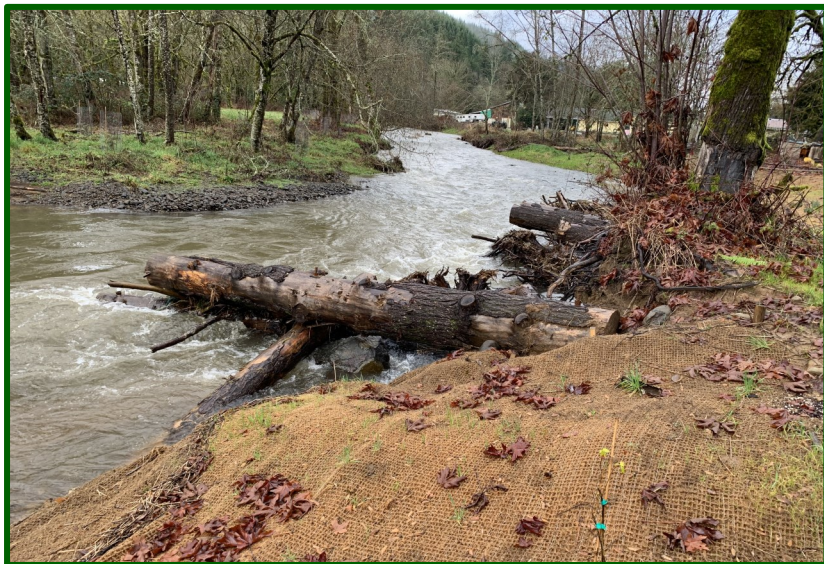
North Scappoose Stream Restoration project. Photo by SBWC, January 2020
