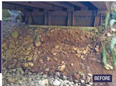
BRIDGE STABILIZATION / SEDIMENT REMOVAL Carcus Creek, Clatskanie, OR
