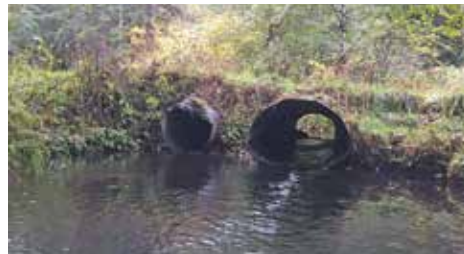
Crossing #5 before construction.
