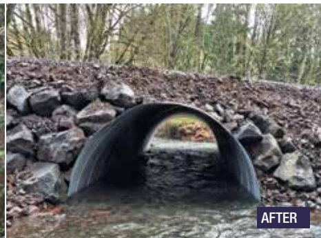
SEDIMENT REMOVAL / CULVERT REPLACEMENT Keystone Creek, Clatskanie, OR
