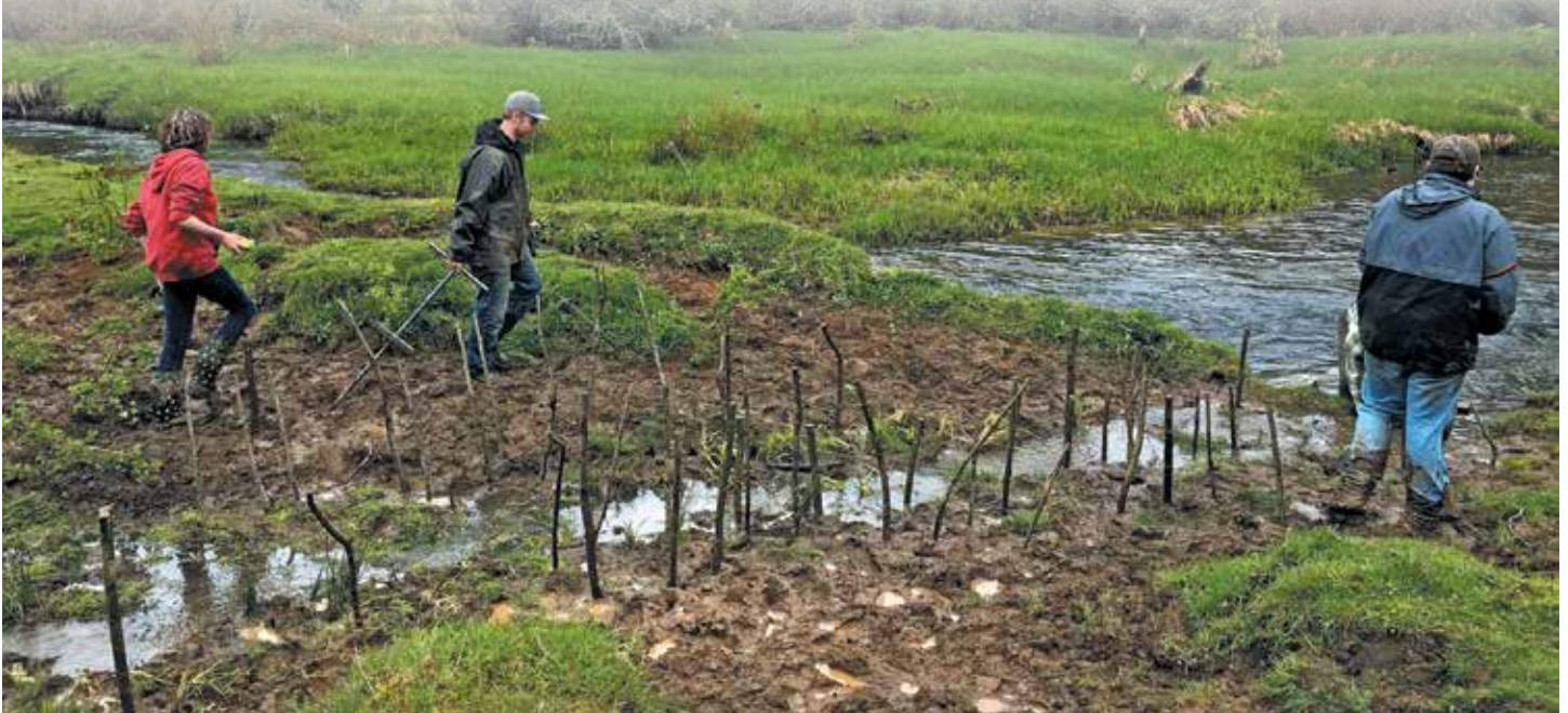
CRYC crew planting willow stakes along a side-channel to improve water quality, soil stability and habitat.
