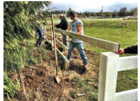
CRYC installing a fence to keep livestock out of the river. This is another important measure in improving water quality.
