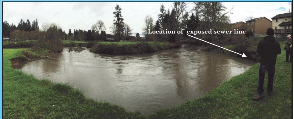
S. Scappoose Creek still close to bankful in March 2016. The channel is C-shaped at this location and heavily incised contributing to the generation of strong and concentrated erosive forces. The lack of a floodplain and vegetation also contributes to erosion.
